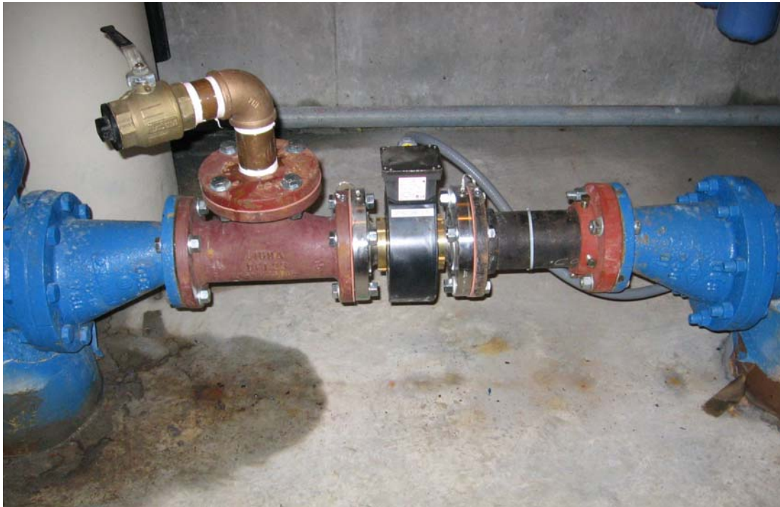
Figure 2. “AquaMaster S” data logger installed at the Alma Aquaculture Research Station. Total accumulated flow and instantaneous flow rate are displayed.
